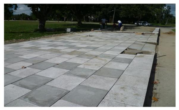
Figure 6. LC<sup>3</sup> pavements at UCLV.
