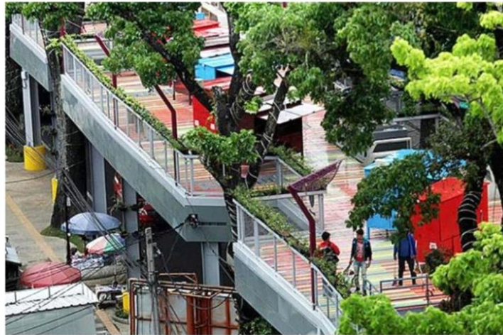
Pic. 4 A special flyover for pedestrians and street vendors called Teras Cihampelas was built on Jalan Cihampelas, Bandung, West Java, and began to be used
