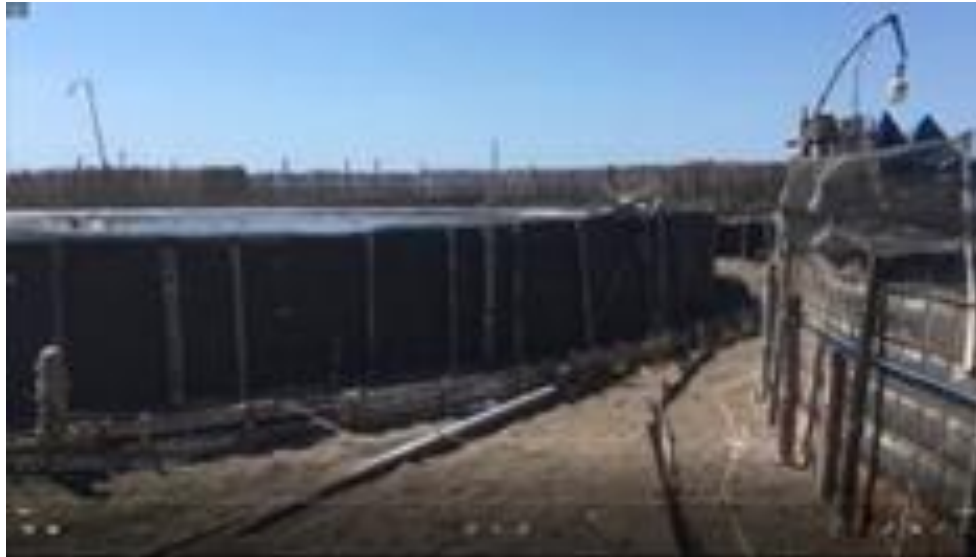
Figure 6: Photo of the condition of the design site
