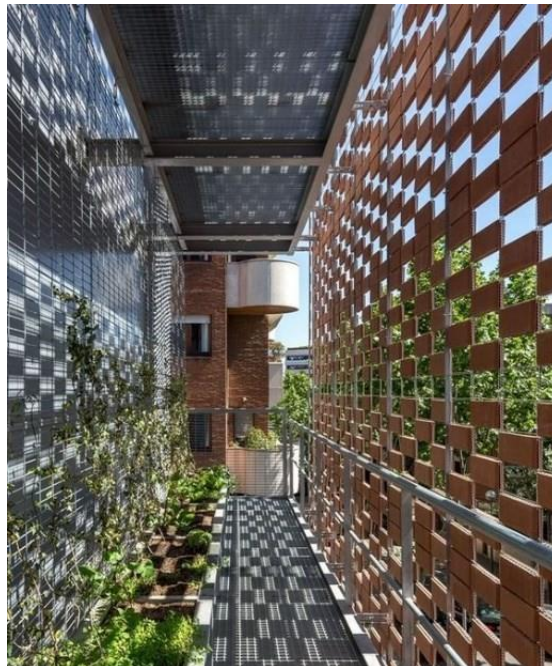
Figure 9. Utilization of Double Facade and Vegetation
