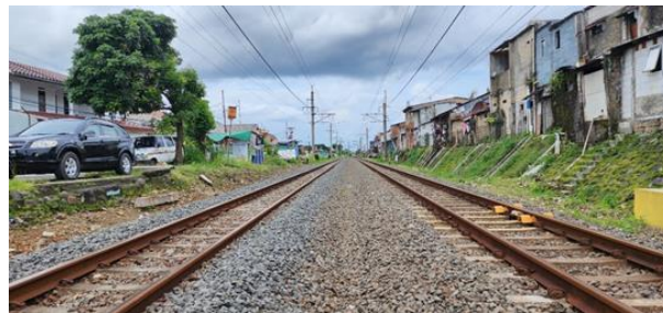
Figure 12. Photo of Differences in Land Leveling
