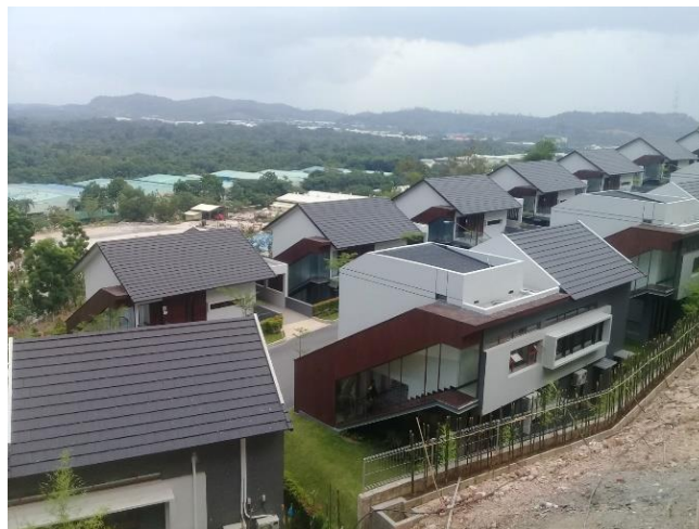
Figure 5 : Roof material : Concrete Tile Source : Writer, 2017
