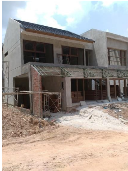
Figure 4 : Walls material : Red brick press Source : Writer, 2017
