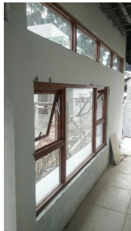
Figure 10 : Opening : Window with balau wood frames
