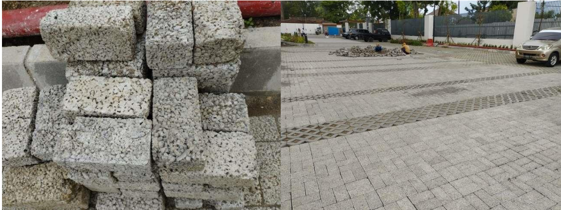
Figure 2: Porous Paving Blocks for the UNU Yogyakarta Campus Building
