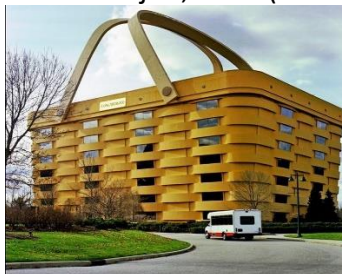
Figure 2: A Basket Building in the United States. Source: Sandler, (2011)
