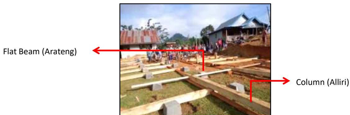
Figure 10. Photo Of Column And Beam Arrangement Source: Personal Documentation
