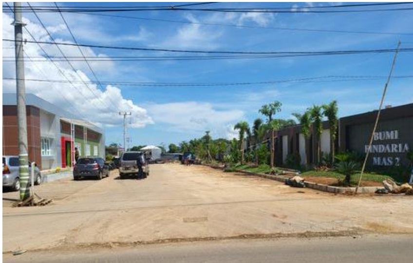
Figure 4. Entrance Gate Bumi Findaria Mas Housing Complex Source: sikumbang.tapera.go.id
