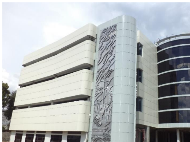
Figure 13. Right side facade Source: Personal Documentation, 2024
