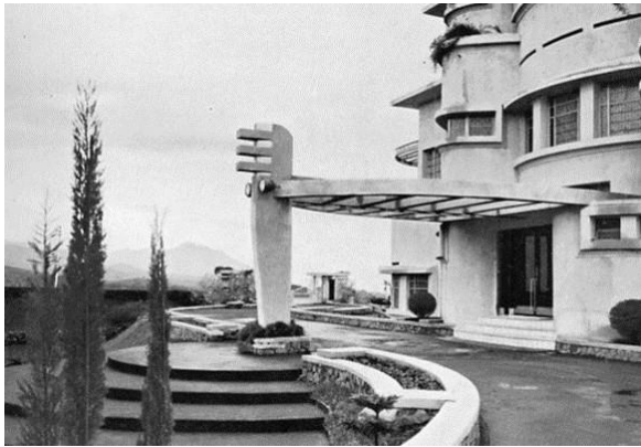
Figure 14. Art Deco style on the Isola Canopy Source: (PT. Daya Cipta Diarancana, 2013b)
