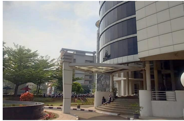
Figure 15. Art Deco style on the Front Canopy (Drop Off) of Mupenas UPI Source: (PT. Daya Cipta Diarancana, 2013b)
