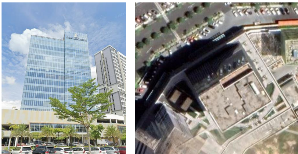
Figure 4. Aria Office Tower Source: PT Citra Buana Prakarsa, 2022
