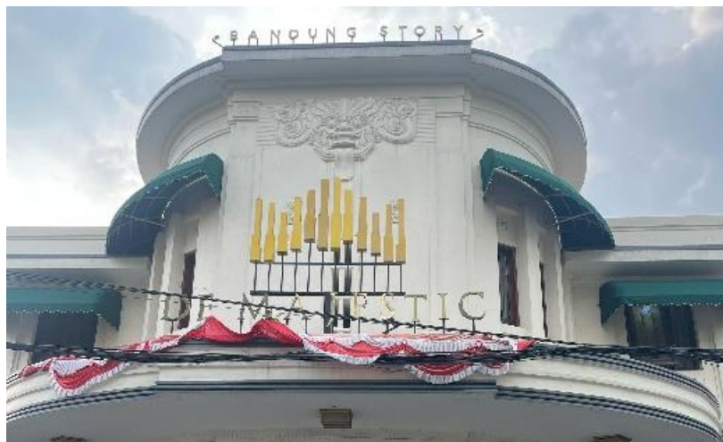
Figure 5. Art Deco style building roof (Source: Author, 2024)
