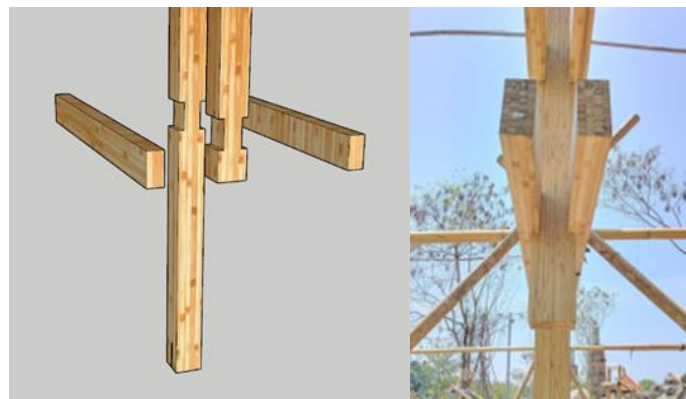
Figure 12. Connection of Laminated Bamboo Columns and Beams (Source: 3D Sketchup and Joint Documents on 1:1 Buildings)
