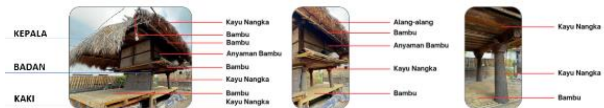
Figure 2. Elements of the "geleng" building with its materials. (Source: Author's survey in 2024)
