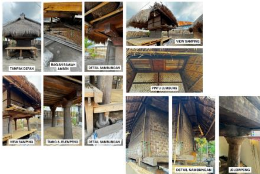
Figure 3. Details of the structural elements of the "geleng" building in Bayan Traditional Village (Source: Author's survey in 2024)
