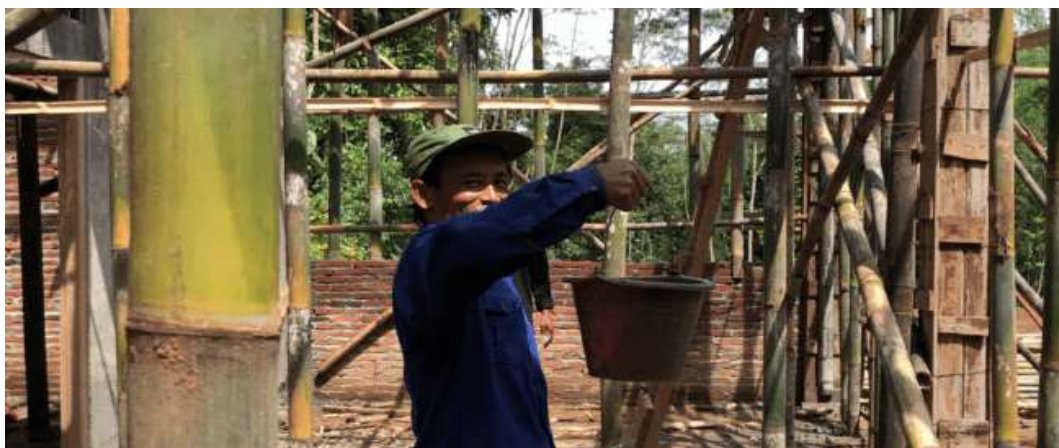
Figure 3: Use of bamboo for concrete supports (Source: Author, 2023)
