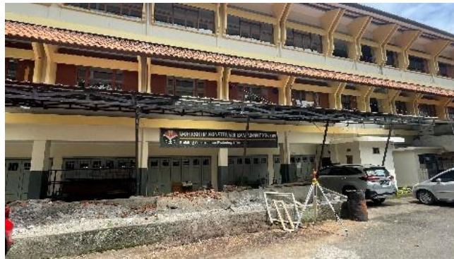
Figure 1. The Entire Facade of Building C FPTI-UPI
