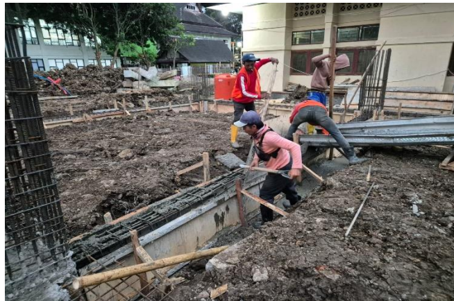
Figure 3. Concrete Footing Work
