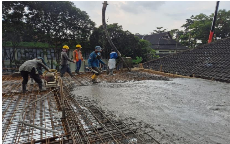
Figure 5. Concrete Work Beams and Floor Slabs
