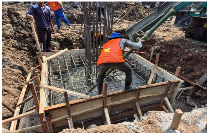
Figure 2. Pile Cap Concrete Work
