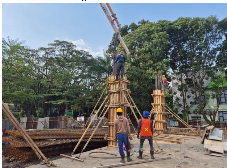
Figure 4. Concrete Column Work
