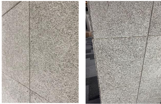
Figure 4 & 5. Materials Used (Wood wool panels) Source: Personal Documentation
