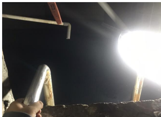
Figure 5. Majesty Apartment Water Tank Source : Private Assets
