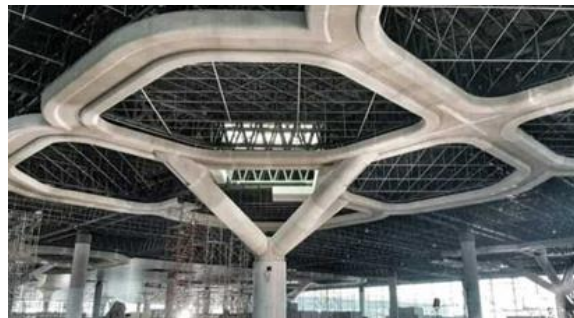
Figure 4.6 Roof Truss Structure of Yogyakarta International Airport (YIA) (Source: https://www.instagram.com/bandarayogyakarta?igsh=ZjhuMGp1cGhtNGRh , 2025)
