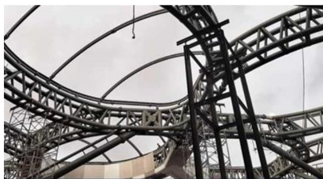
Figure 4.3 Roof Truss Structure of Yogyakarta International Airport (YIA) (Source: https://www.instagram.com/bandarayogyakarta?igsh=ZjhuMGp1cGhtNGRh , 2025)
