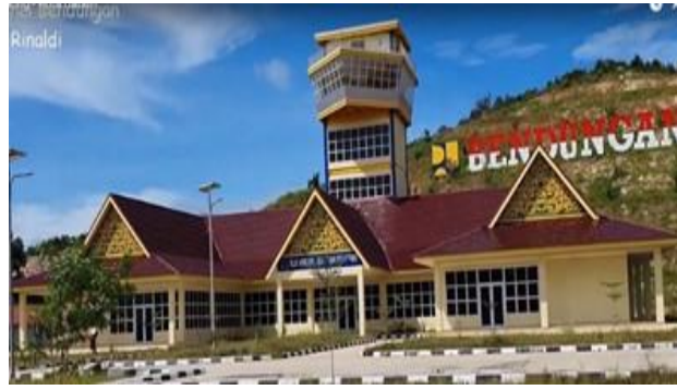
Figure 1. Exterior view of the Dam Management Building. Source: Instagram @arisandruo, 2020
