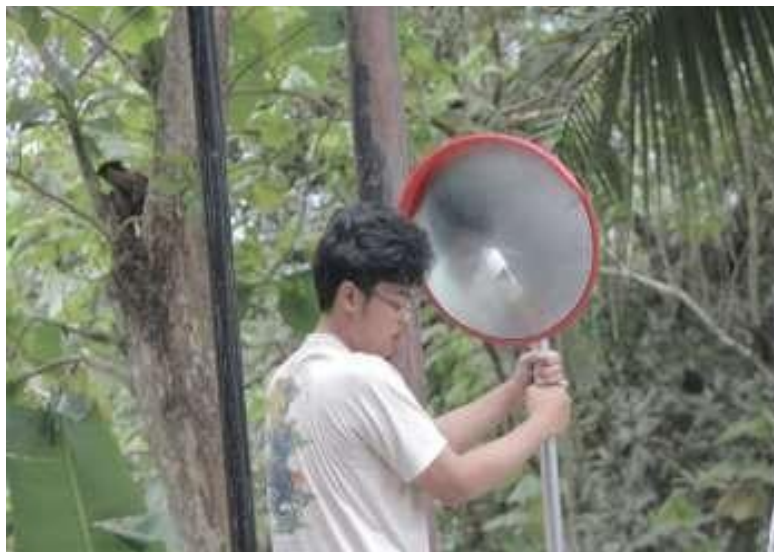
Figure 2. Process of installing a convex mirror Source: Author Documentation 2023
