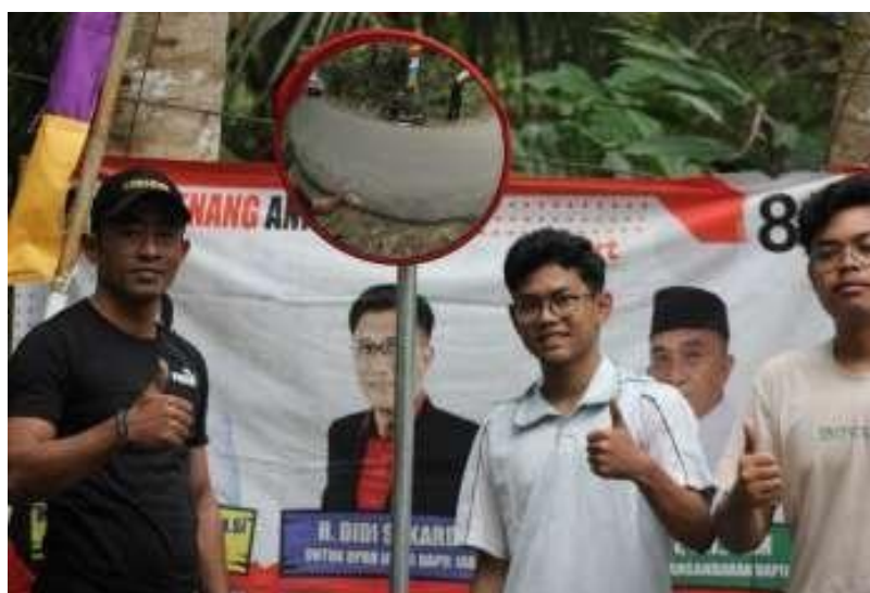
Figure 3. Installation of a convex mirror accompanied by the Head of Bengkekan Hamlet Source: Author Documentation 2023
