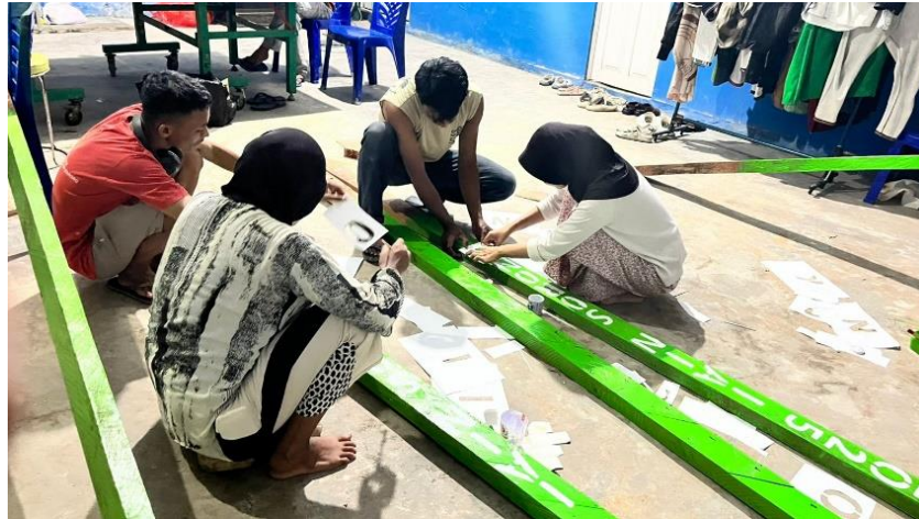
Figure 1. Streetlight Construction Source: Documentation, 2025
