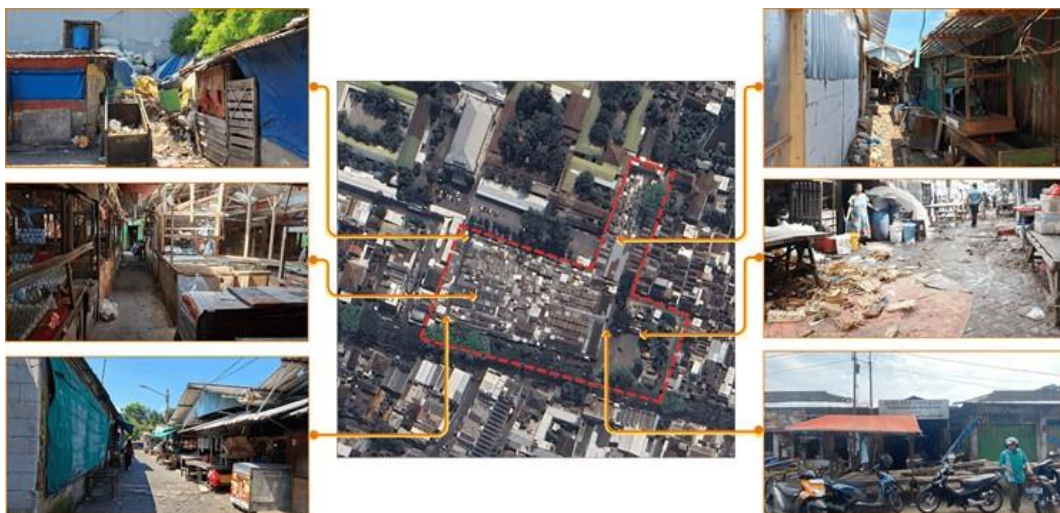
Figure 3. Existing Condition of Blimbing Market, Malang City (Source: documentation, 2026)
