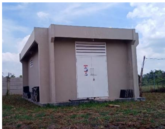
Gambar 4. Ruang genset di Tropical Valley Sumber: Pribadi
