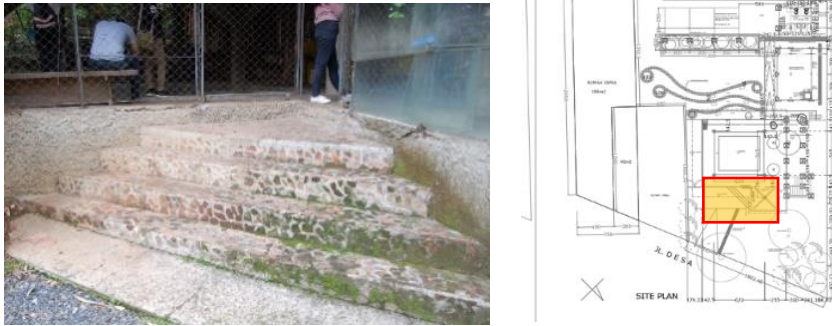
Gambar 6 Material Lantai Batu Alam Area Main Entrance Studio Akanoma (Sumber: Data Studio Akanoma & Data Pribadi)
