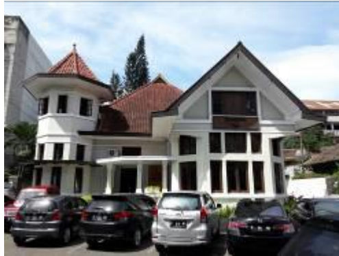
Gambar2. Facade Dakken Restaurant
