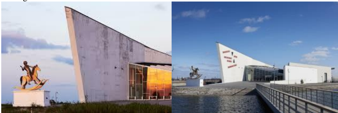
Figure 1 Exterior of Arken Museum Source: (Team, 2017)
