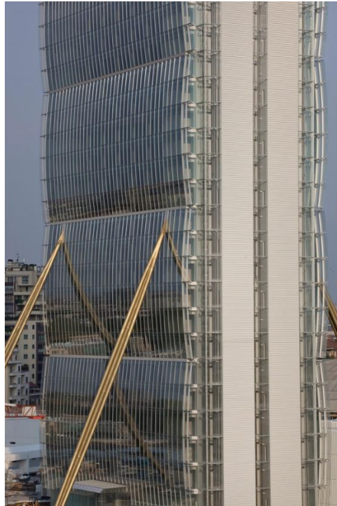
Gambar 8. Fasad Allianz Tower Sumber: ArchDaily, 2015
