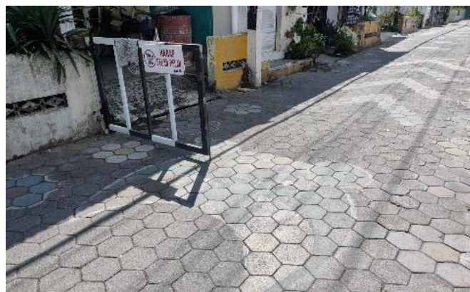
Figure 13. Street Material Using Only Paving Blocks (Source: Personal Data, 2024)
