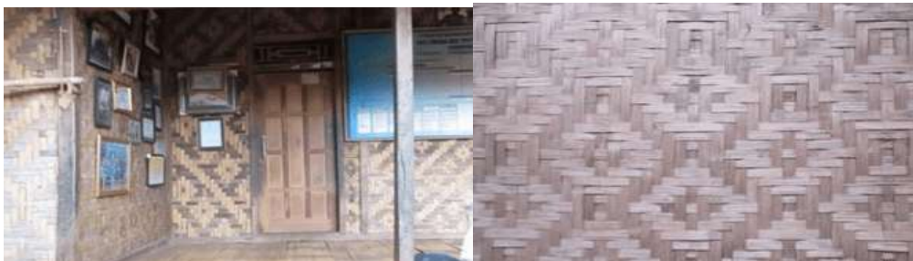
Figure 14: Woven Bamboo Wall (Source: Harapan, 2019)
