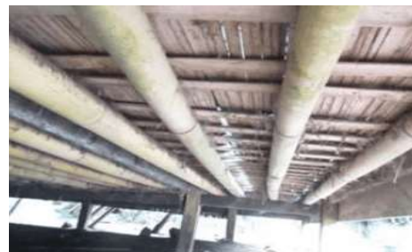
Figure 16. Bamboo Floor Support (Source: Harapan, 2019)
