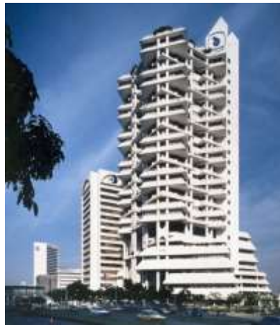
Figure 1.1 Wisma Dharmala Building
