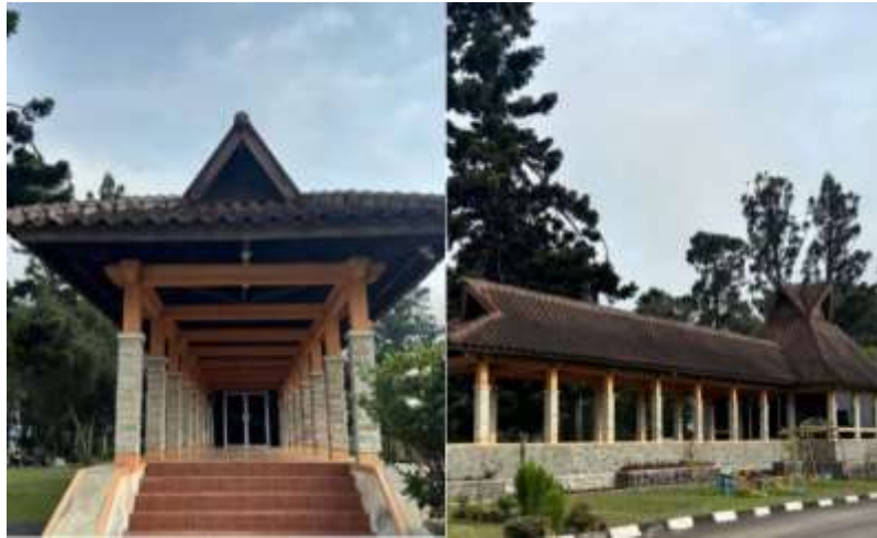
Figure 9. The shape of the Julang Ngapak roof (Source: Personal Documentation, 2024)
