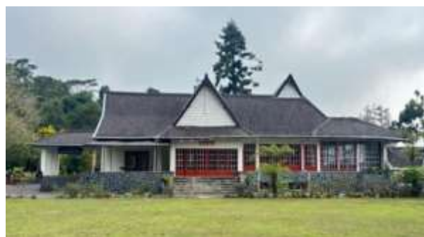
Figure 1. KAR Bosscha House Building (Source: Personal Documentation, 2024)
