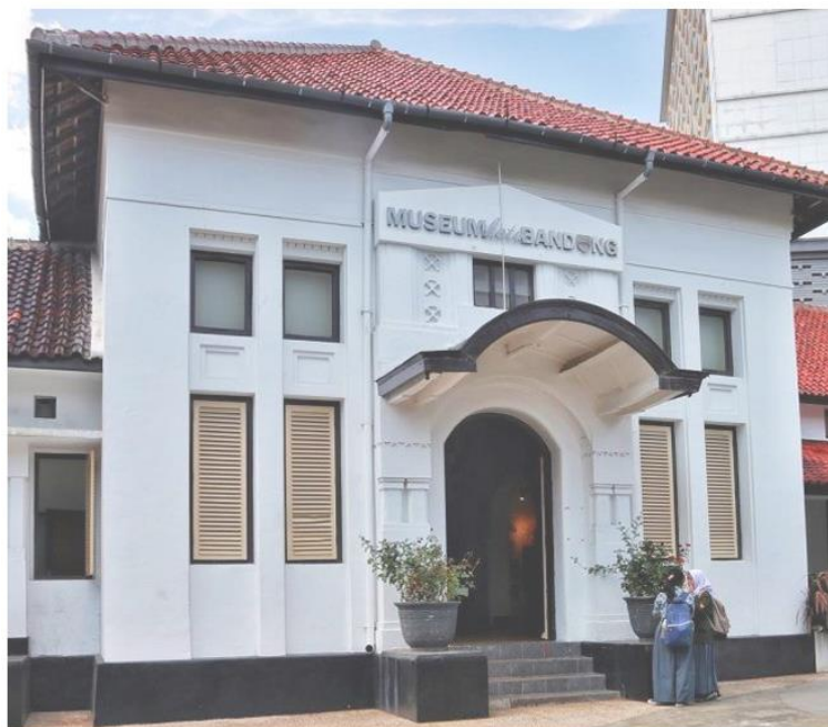
Main Door of Building Image
