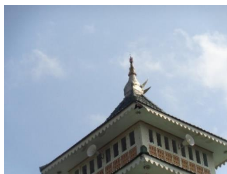
Figure 8: Momole on a multi-pitched roof (Source: personal document, 2024)
