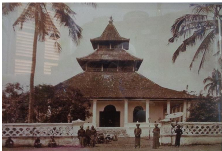
Figure 3: Manonjaya Grand Mosque in 1832 (Source: Personal Data, 2024)
