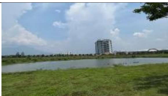
North retention pond in Summarecon Bandung
