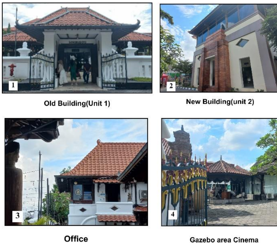
Figure 9. Roof Shape (Source: personal documentation, 2025)
