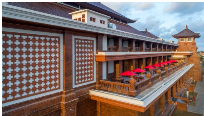
Figure 6. Building Details of Balai Budaya Giri Nata Mandala (Source: PT. Tunas Jaya Sanur, 2025)
