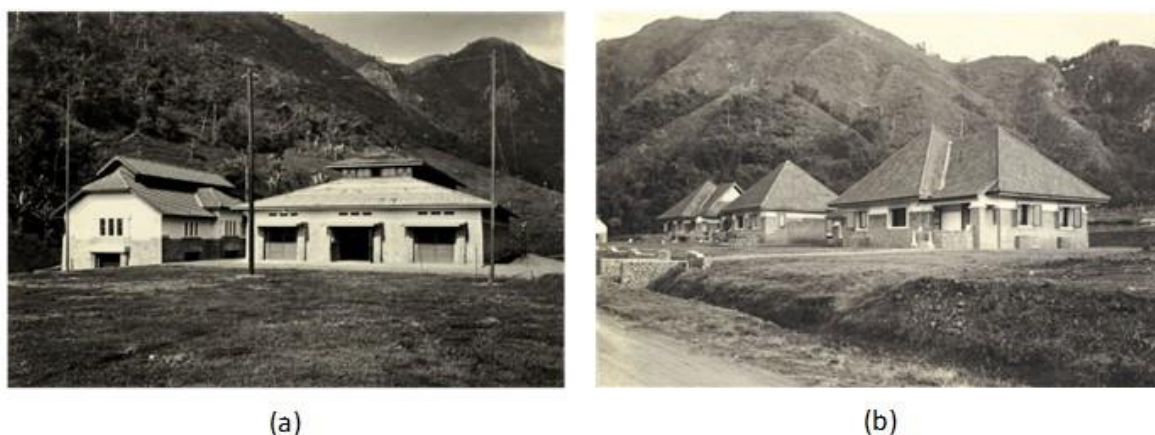
Figure 4. (a) Radio transformer building (left) and transmitter building (right) (b) Official residence (Dientswoning).
