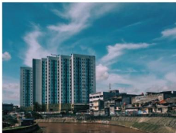
Figure 3. Modular Facade of Rusunawa Jatinegara Barat Source: Author, 2019
