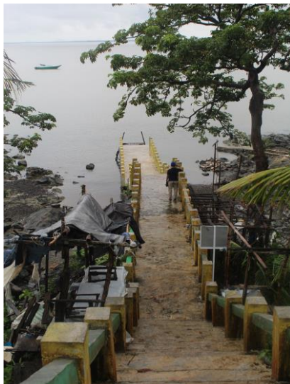
Figure 3. Piers of Pulau Datu Island (Source: Author, 2025)
