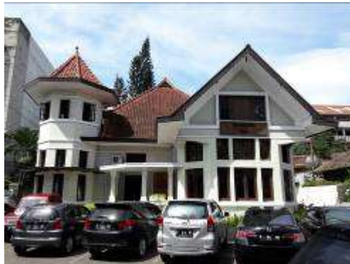
Gambar 3 Facade Dakken Restaurant
