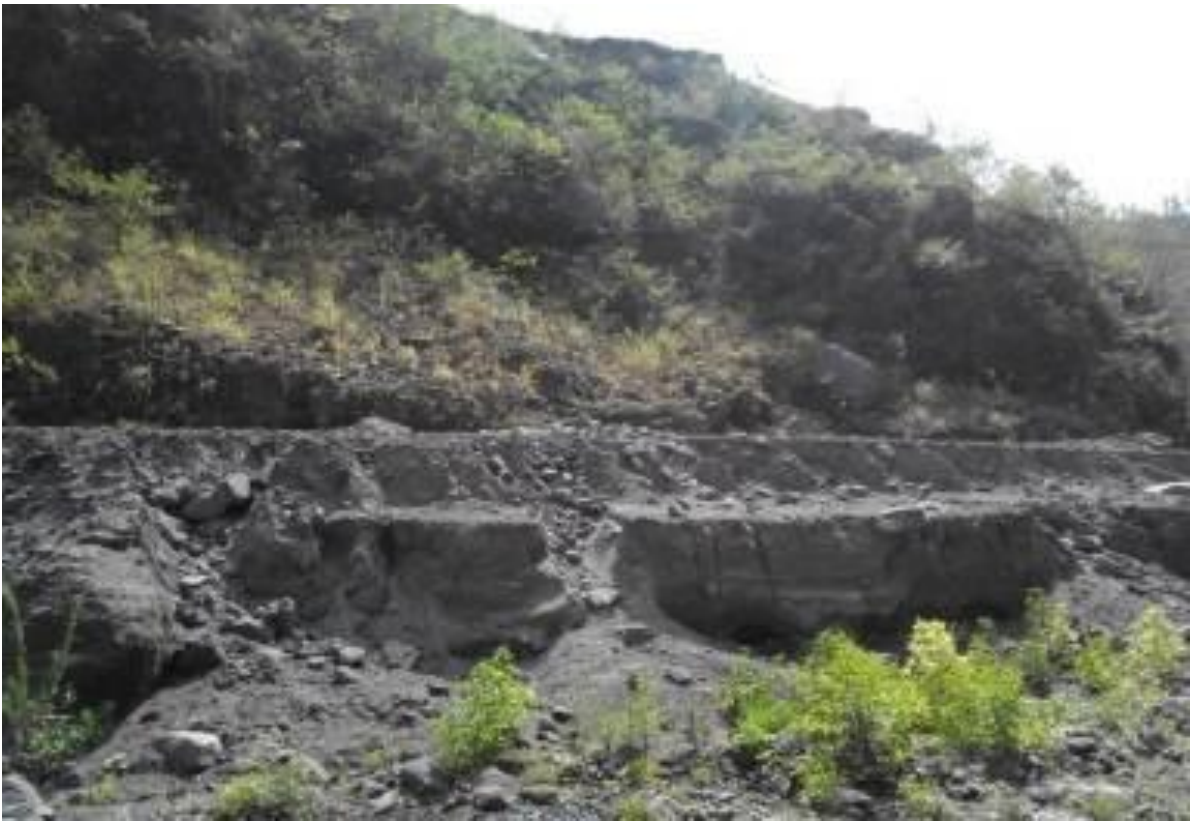
Figure 6. Lahar deposits along the base of riverbanks (Photo: Handayani, 2014)
